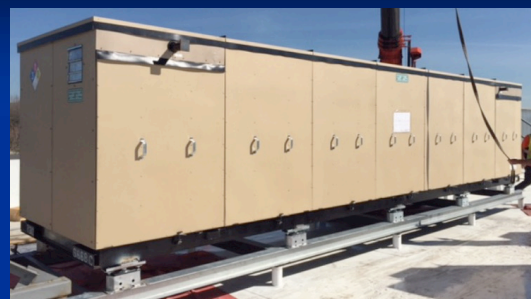
PACKAGE CHILLER ON ROOF TOP
