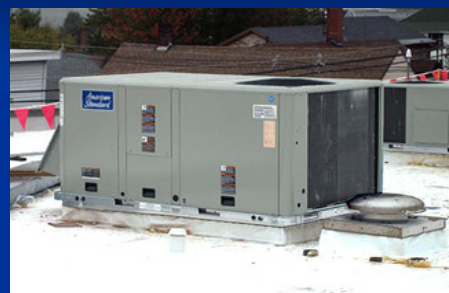
Package Ammonia Chiller Installed on roof top
