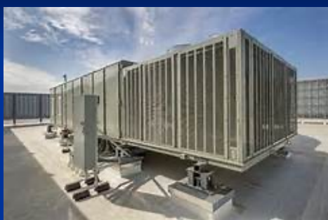
Package Ammonia Chiller installed on Roof Top
