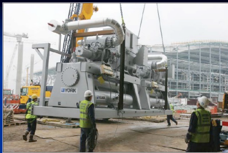
One of The Four package Ammonia Chillers being installed at Heathrow Airport
