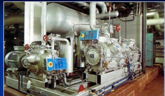
The complete Ammonia Chiller package including electric starter panel and all wiring at the P&T building, Copenhagen.
